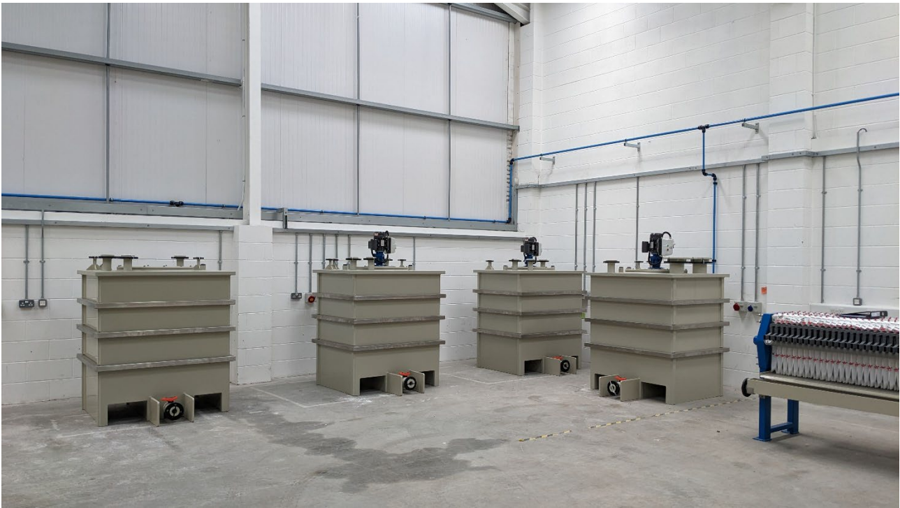
Figure 2: Process Reactors in position adjacent to installed utilities and services.
