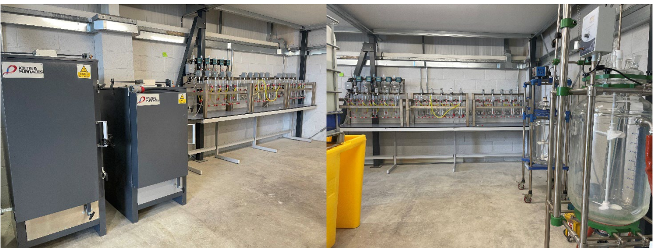
Figure 9: Pilot plant relocated to new mezzanine area; left, demagnetisation oven and product drying kilns, and right showing glass reactor arrangement adjacent mixer-settler circuit.
