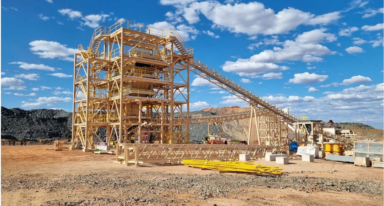
Figure 3: Structural steelwork at the screen deck as at 26 March 2023.
