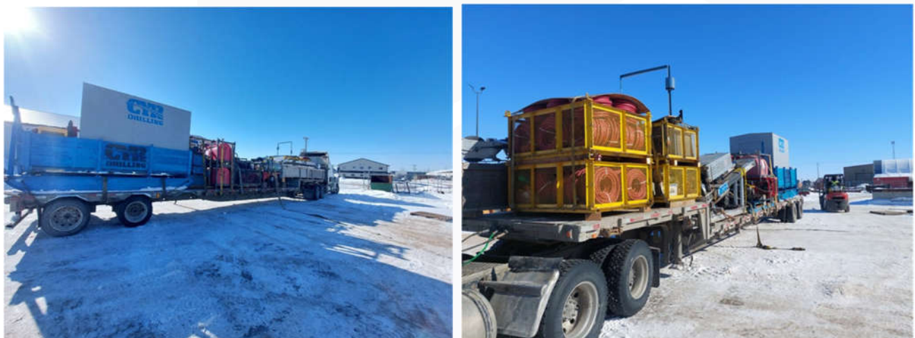
Figure 8 – Mobilised drill rig equipment and supplies
