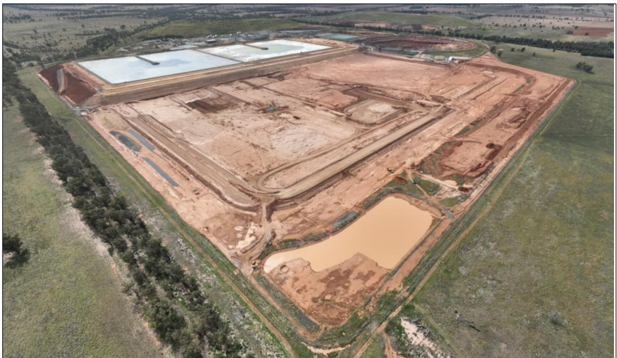
Residue Storage Facility 2 under construction
