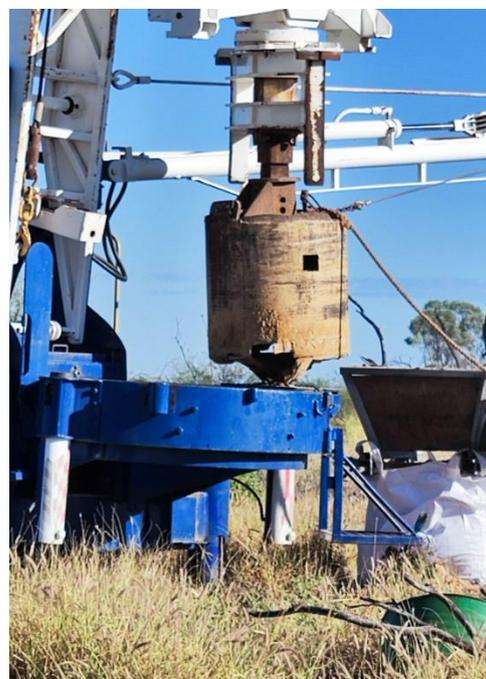
*Photo 1. Caldwell bucket rig with 900mm diameter bucket, and hopper for safe and efficient loading of bulk bags*
