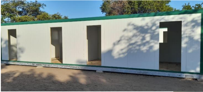
Figure 6 - Accommodation Unit (External)
