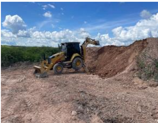
Photos 1 and 2: Drill pad preparation, at top of Bom Jesus de Baixo mine (left) and at second pegmatite outcrop (right)
