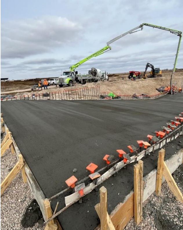
Figure 3. Longs Peak Dairy- fluid retention basin floor.
