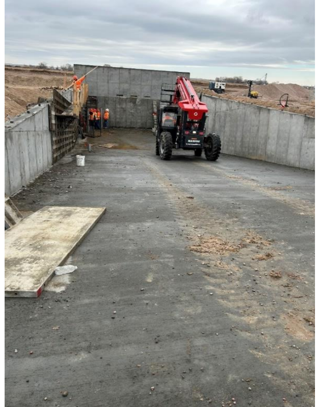
Figure 4. Longs Peak Dairy-fluid retention basin with walls.
