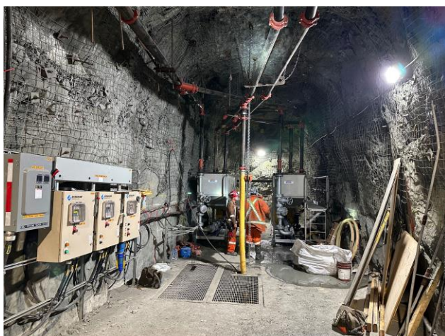
Figure 4: New Sugar Zone pump station installation, improving pumping capacity, reliability and reducing dewatering cost
