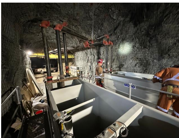
Figure 4: New Sugar Zone pump station installation, improving pumping capacity, reliability and reducing dewatering cost
