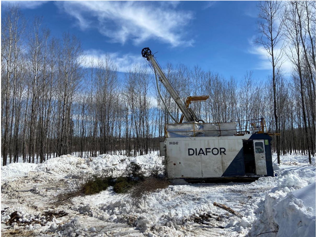
Photo 1: Diafor Drilling Rig in Operation at Chubb Lithium Project Site
