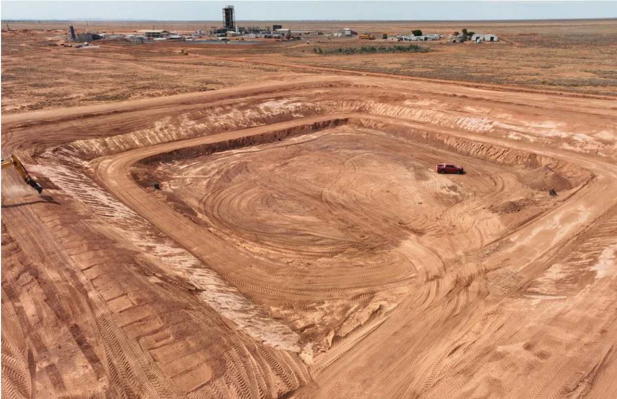
Image 5: 60,000 cubic metres excavation earthworks for the 25,000 ton gypsum pond now complete
