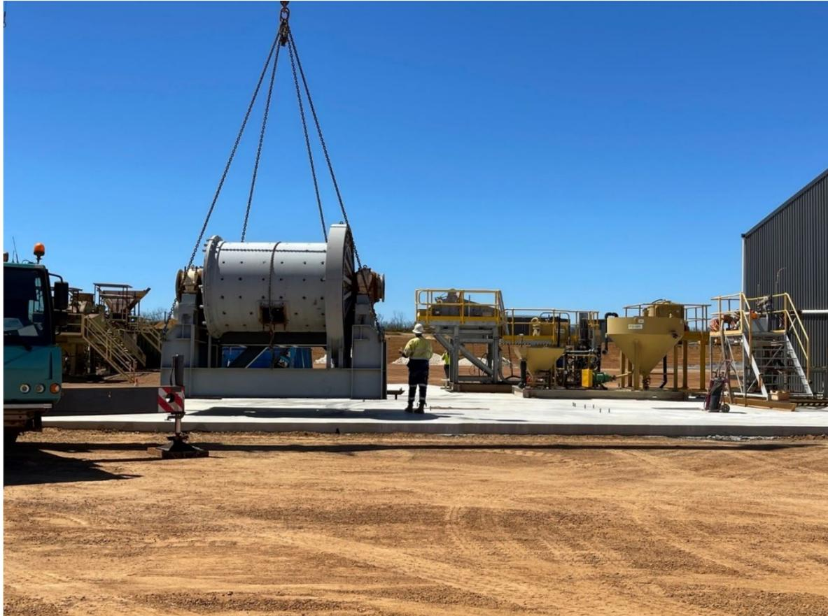
**Figure 12: Picture showing Ball Mill, Trommel and water tanks.**
