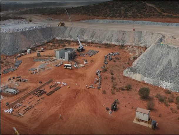
Figure 7: Run-of-Mine pad with primary crusher foundations
