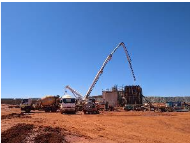
Figure 5: Pouring of the Fine Ore Bin foundations
