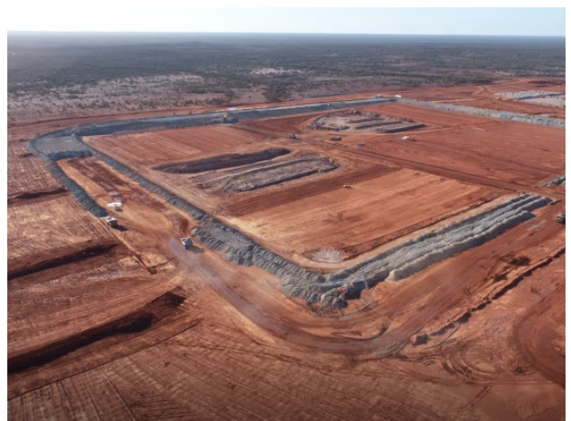
Figure 4: Tailings storage facility
