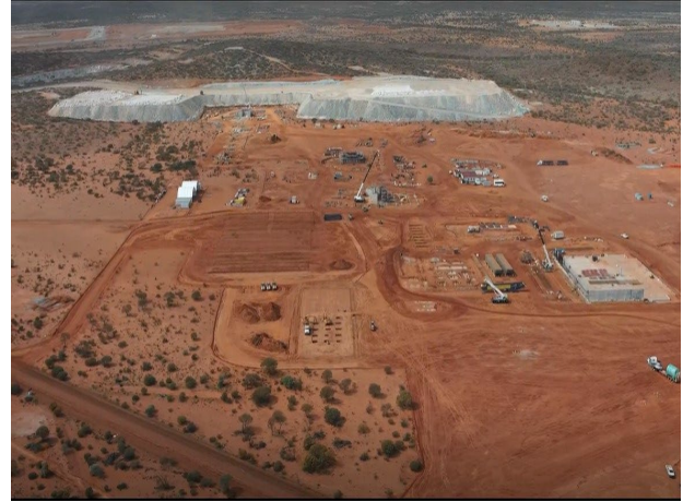
Figure 8: View of the Run-of-Mine pad and processing plant footprint
