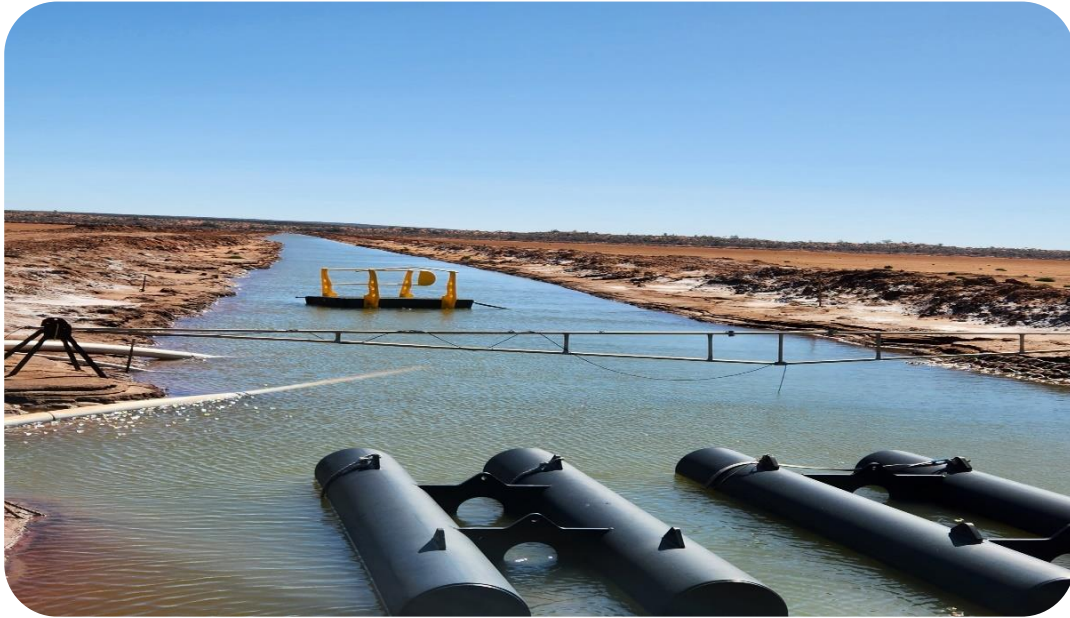
Lake Sunshine trenches, March 2023
