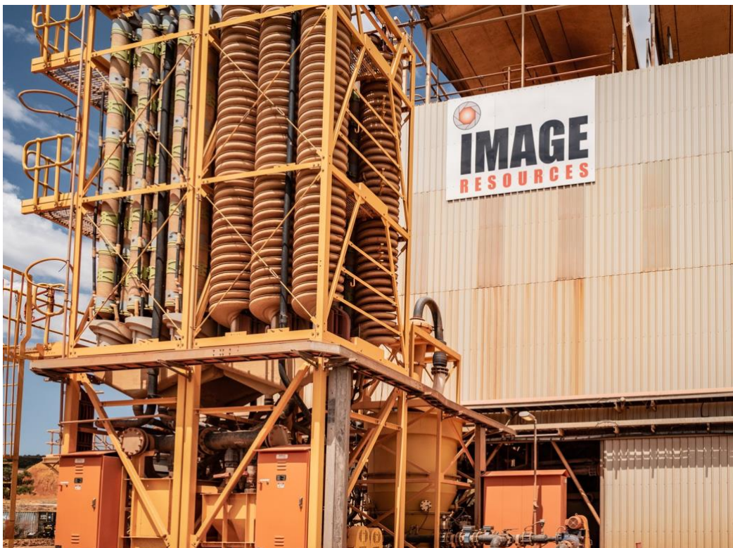
Photo 1: CT1 Demonstration Plant at Boonanarring
