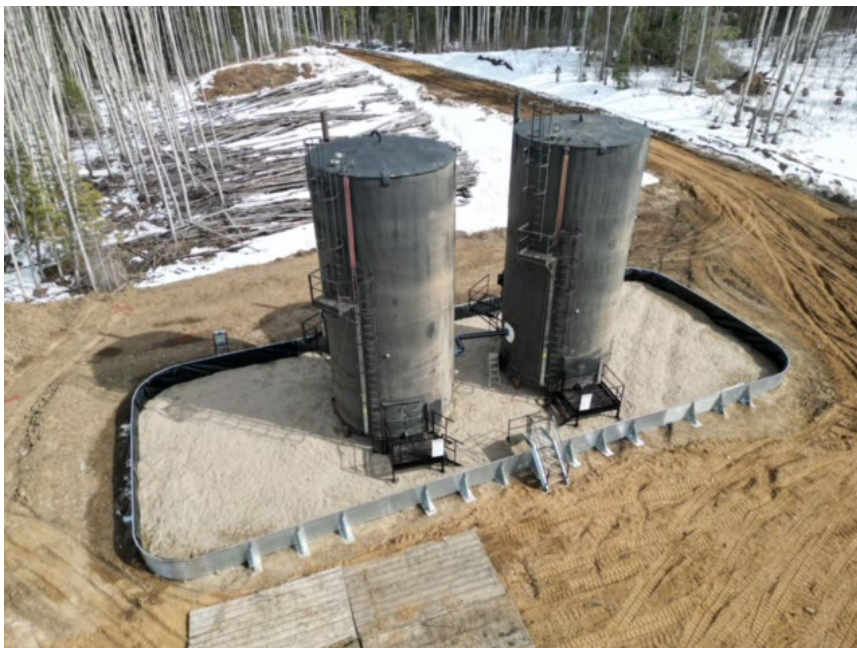
1000 Barrel Storage Tanks at one the new wells
