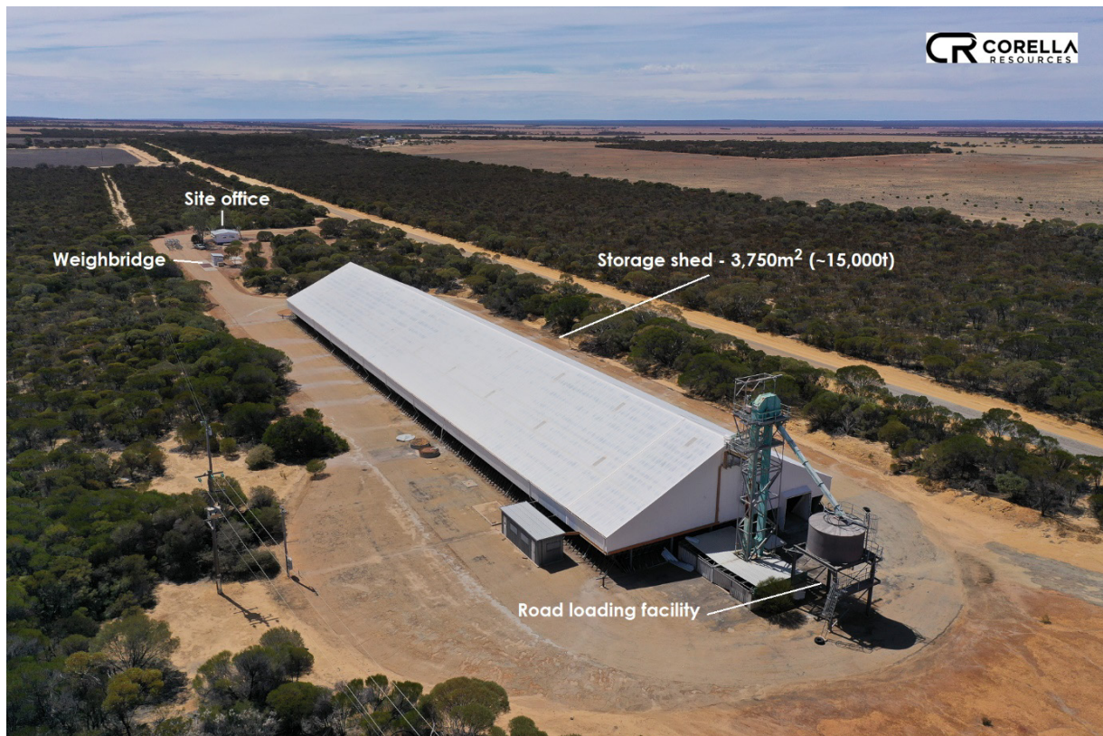
Figure 9: Tampu storage facility (view looking NNE)
