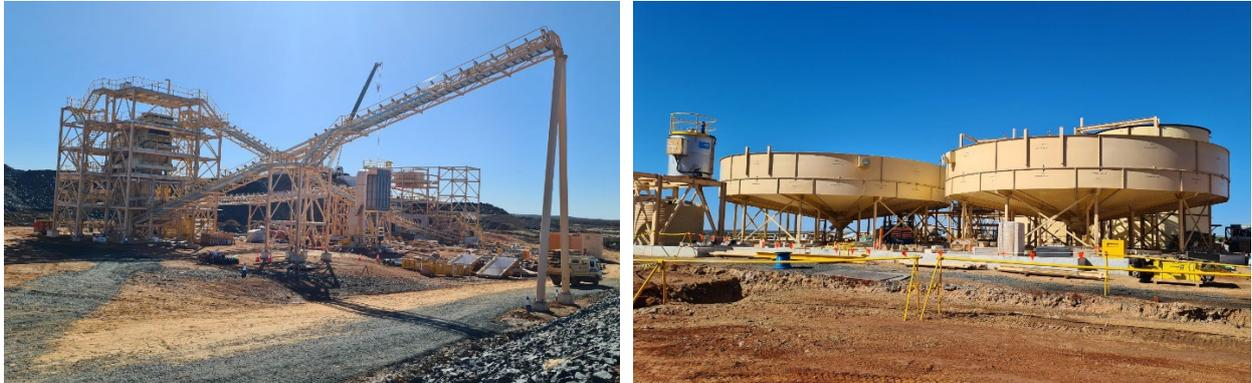
**Figure 7:** Construction progress on site at the end of April 2023 with partially painted CIL tanks, structural steel work well advanced on the crushing and screening areas and fine ore bin construction commenced.
