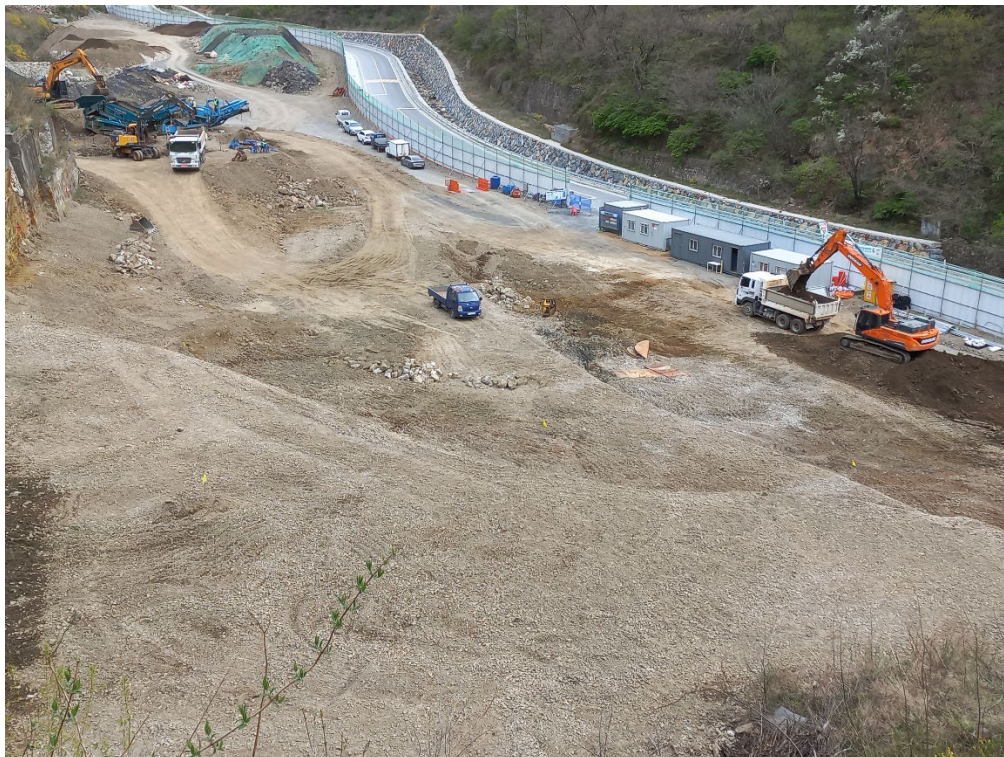
Surface Scalping at the Sangdong Tungsten Mine site, with Temporary Site Offices, New Roads and Drainage in the Background.
