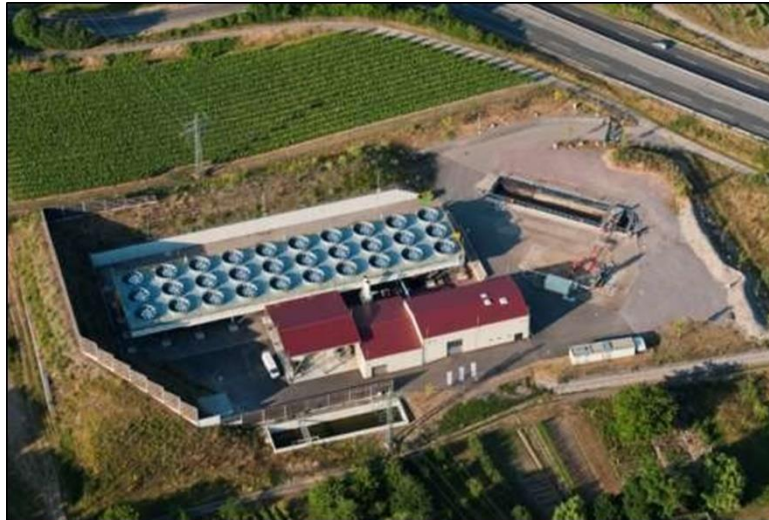
Figure 3.4: Aerial photograph of the Insheim Geothermal Plant. Source Pflazwerke Gruppe (2019).
