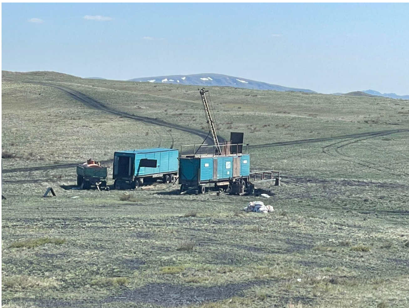
Figure 1 – Geotechnical Drilling at the Sarytogan Graphite Deposit, Central Kazakhstan.
