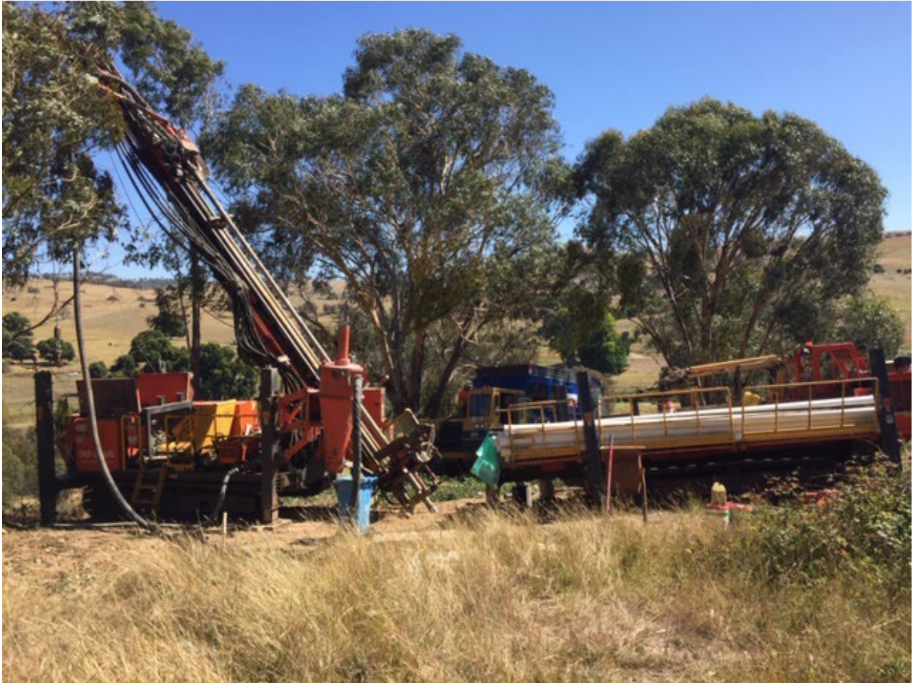
Figure 2: Drilling commences at the Perkins West Deposit at Gibraltar in early March
