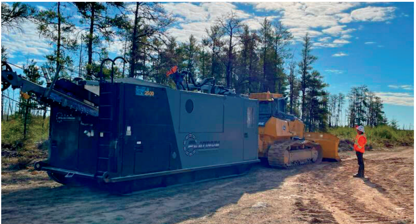
Figure 1 Platinum Diamond Drilling rig onsite at William Lake Nickel Project.
