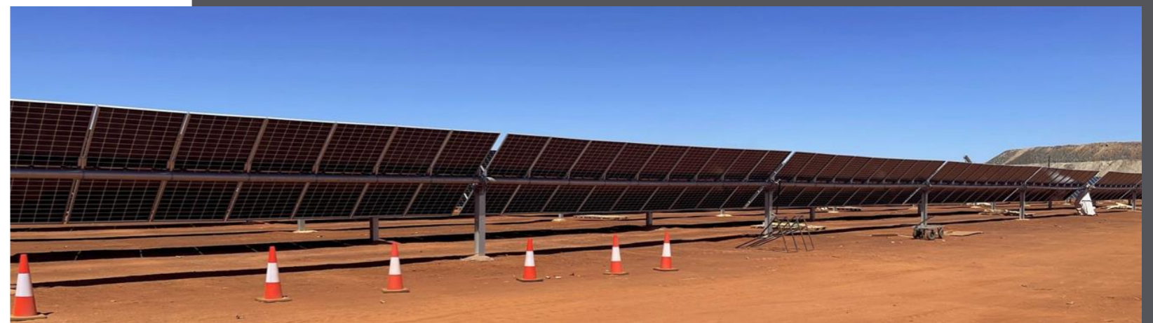
Installation of 9MW solar farm (Duketon)
