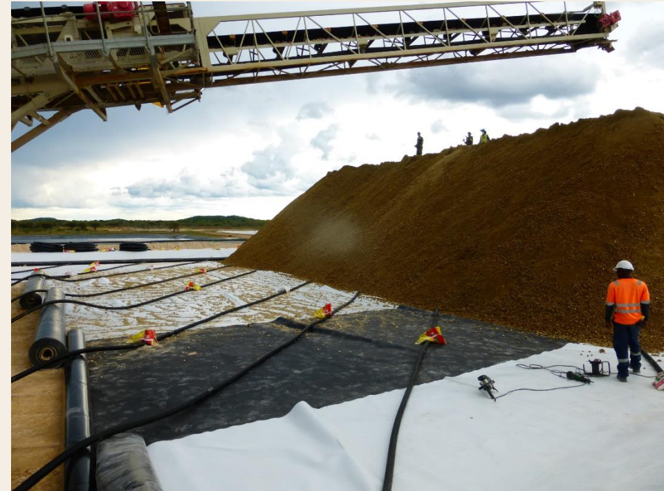
Figure: Example of Heap Leach construction
