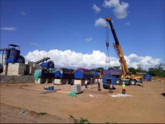
Figure 2: Lifts of the flotation cells onto their plinths on the lower section of the concentrator building. Note the lift of the last floatation cell in the picture on the right.
