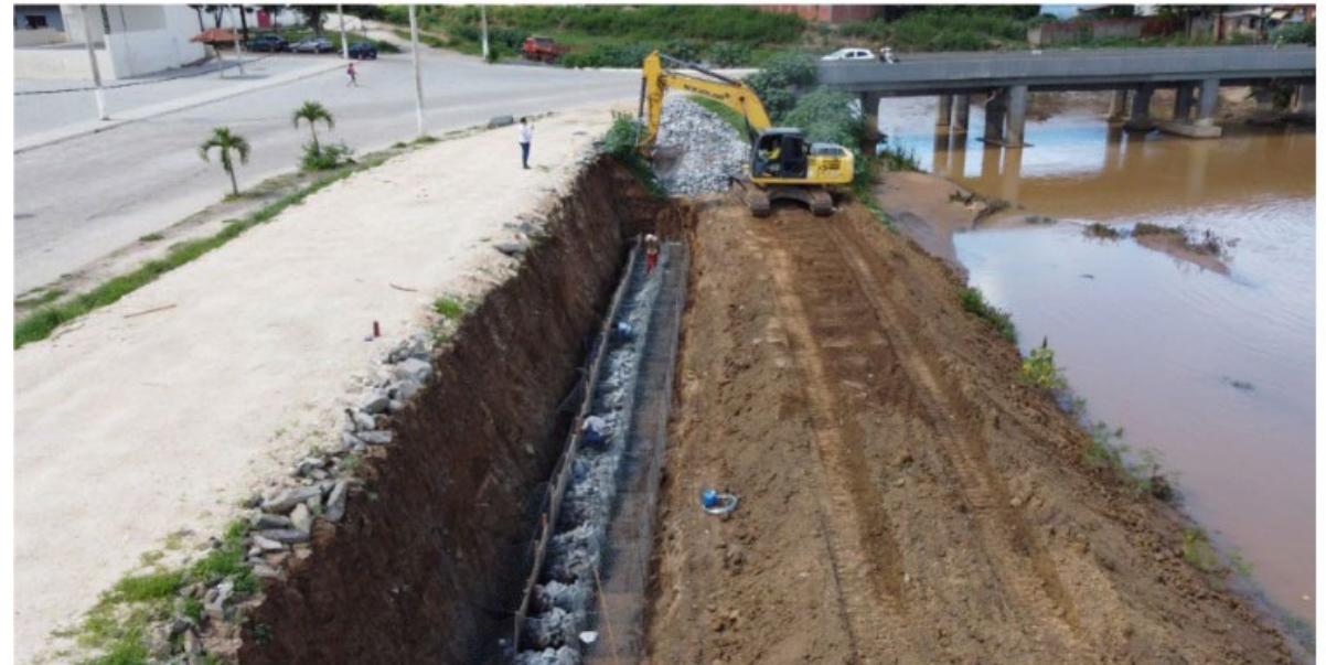
LRS funded levy wall in Salinas built December 2022
