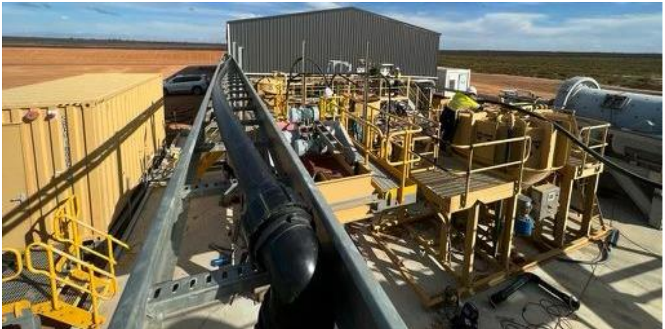
Figure 2: Kat Gap GEKKO PROCESSING PLANT.
