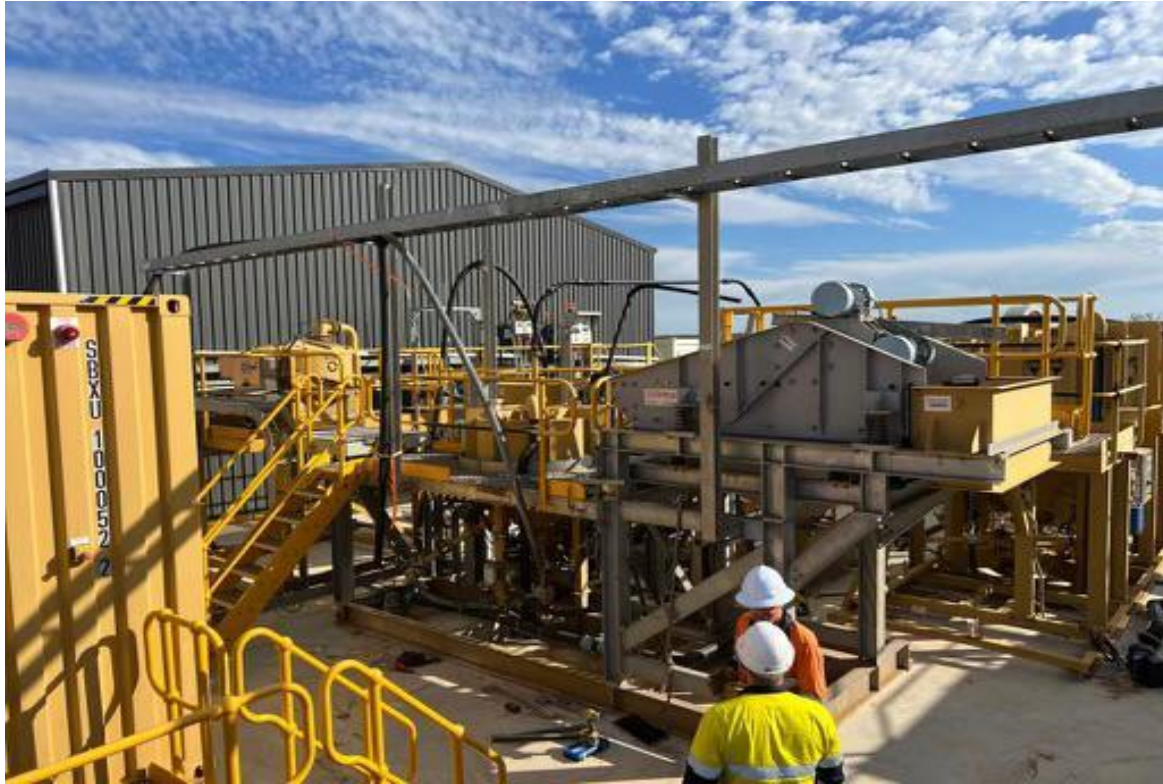
Figure 3: IPS staff working on the plant.
