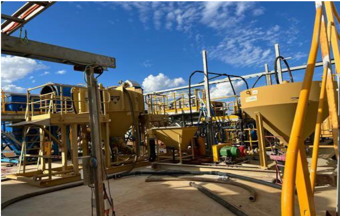
Figure 1: Kat Gap GEKKO PROCESSING PLANT.
