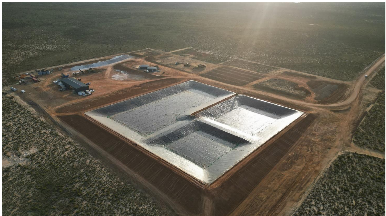
Figure 4: TSF with lining completed in April 2023.
