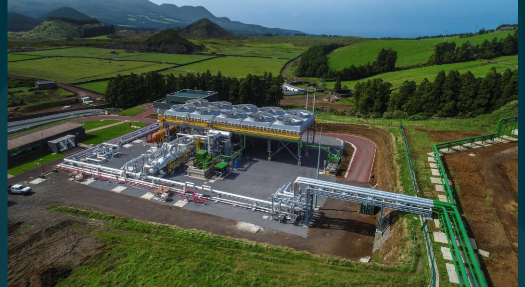
Pico Alto Geothermal Plant, Azores. Courtesy of Exergy International Srl
