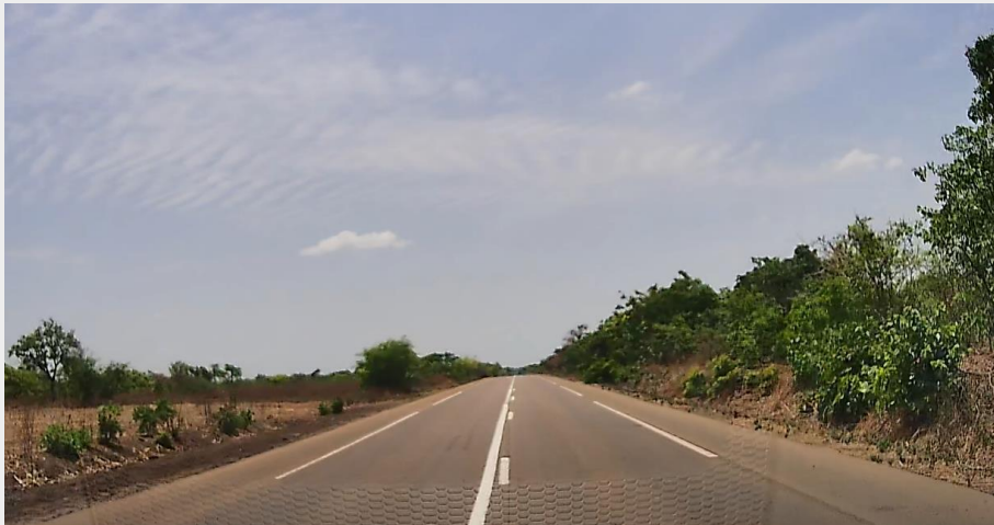
Typical road condition - Tingrela area
