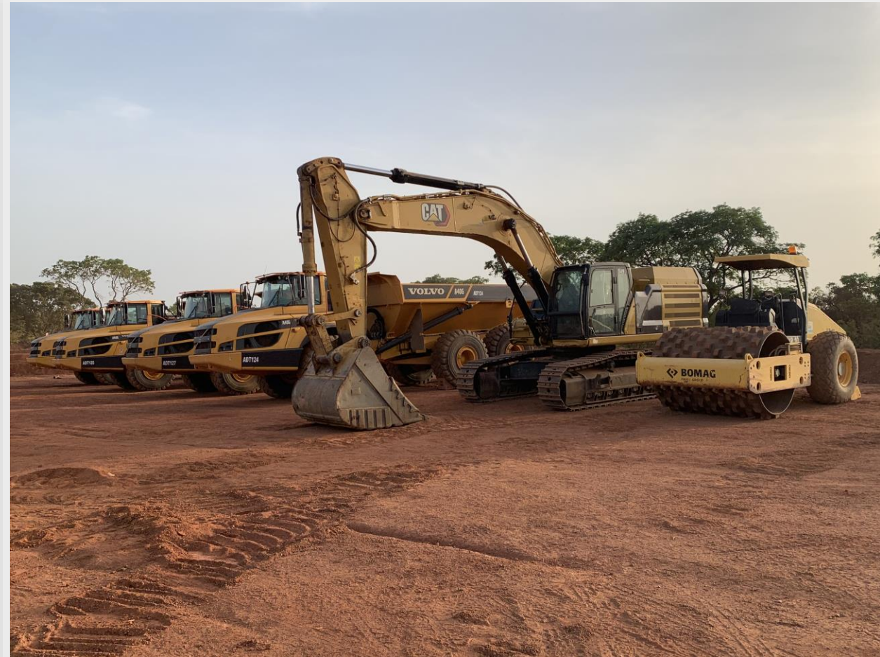
Mobile equipment fleet started arriving in late April
