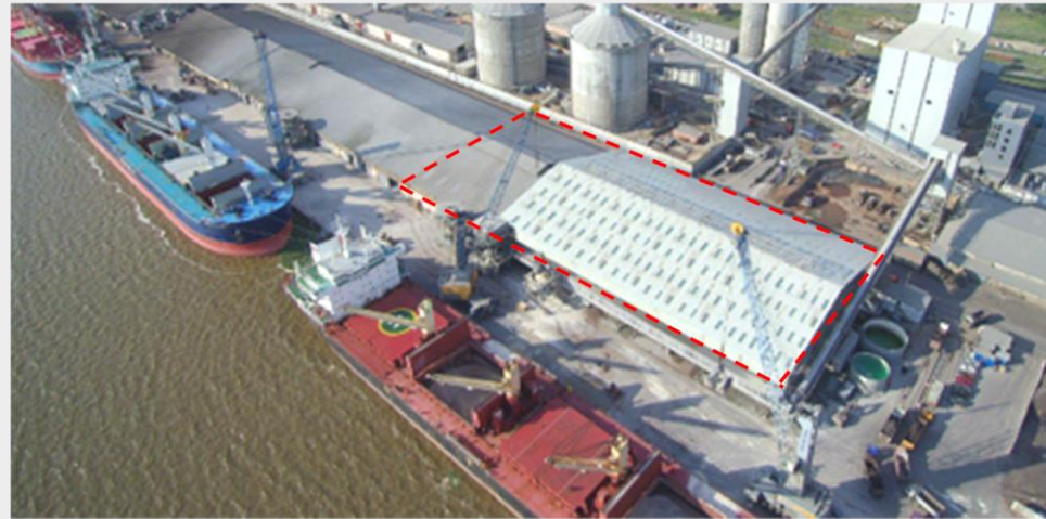
Abidjan Port bulk export loading facility and secured warehouse
