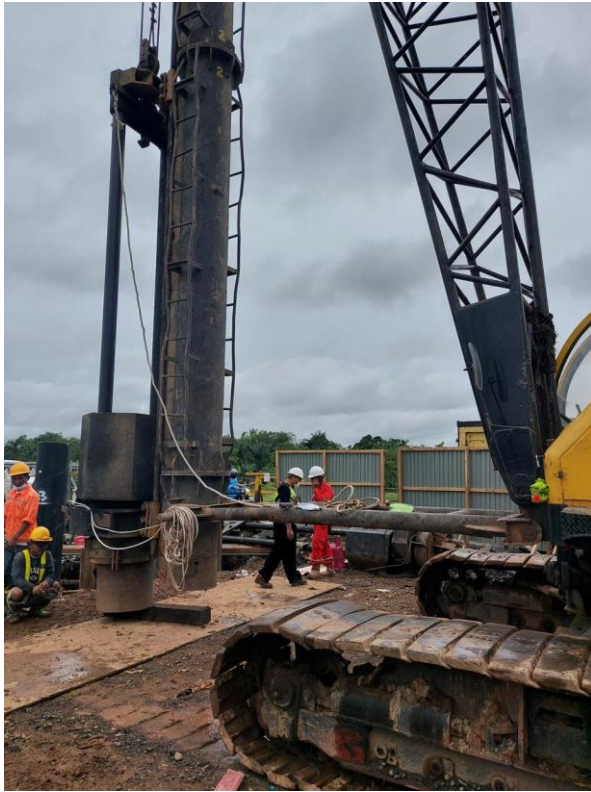
Photo: Piling Crane
