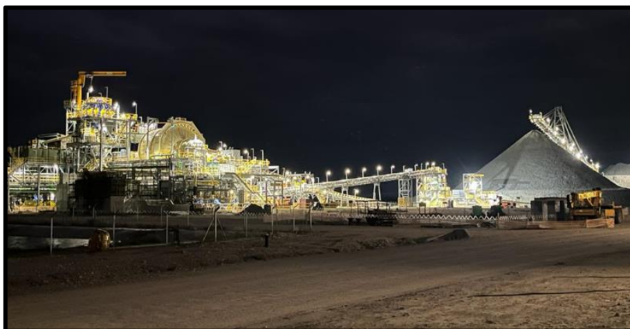
Figure 1: Motheo Copper Mine Process Plant.
