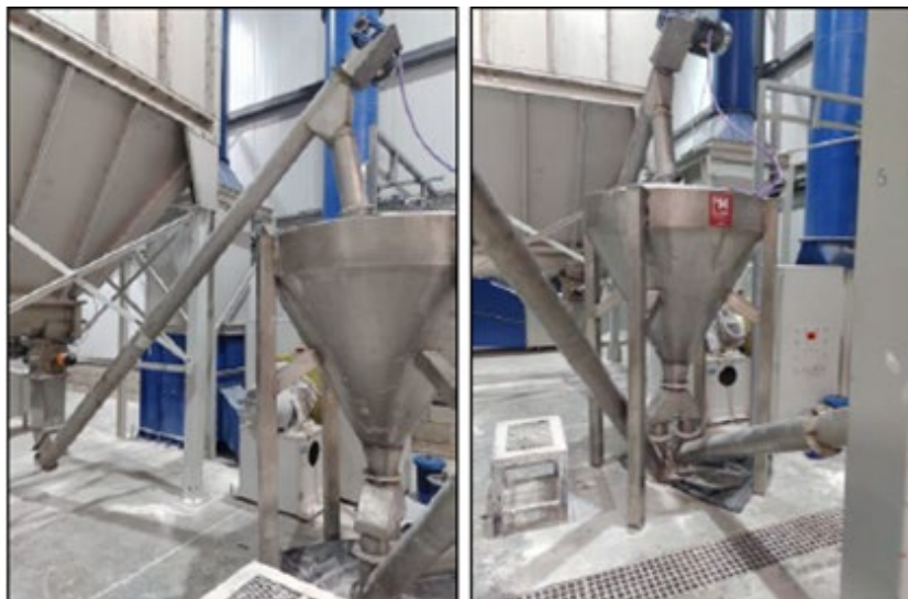
Figures 7-8. Rincon Lithium Project – 2,000tpa Operation Commissioning Works
