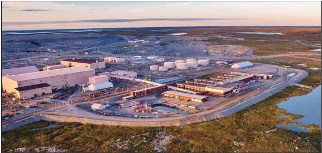
Figure 1-1: Ekati Diamond Mine main infrastructure
