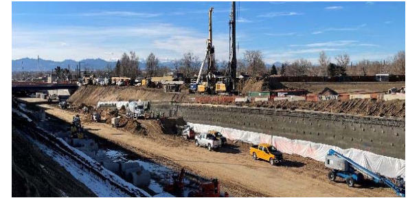
I-70 Shotcrete project in Denver
