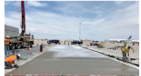
Denver Airport- concrete replacement -United Airlines
