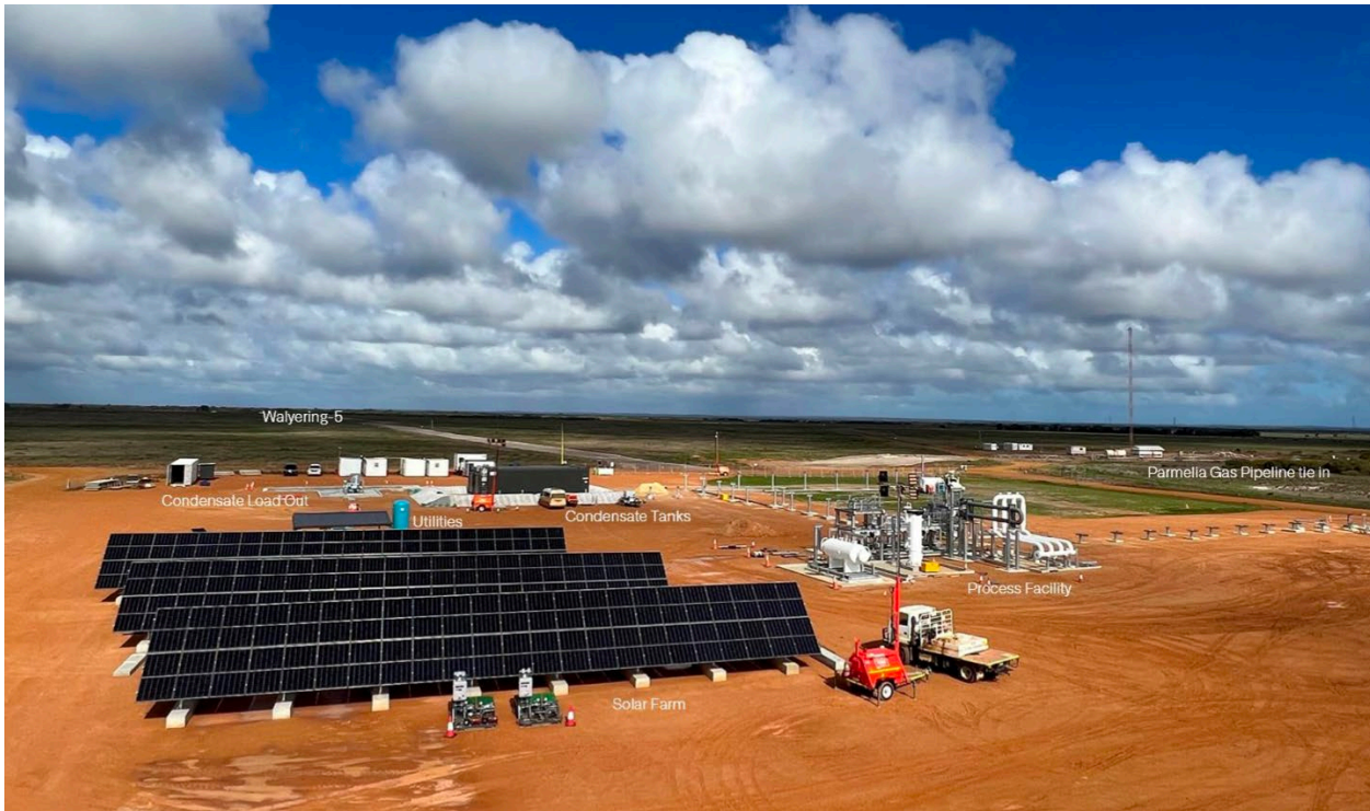
Figure 1 – Bird’s-eye view of the Walyering Production Facility (image provided by Strike Energy)
