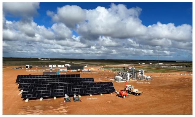
Since the last update Strike has continued construction at the Walyering gas field which has progressed without incident and in line with its revised schedule. All processing equipment is now secured in place, condensate tanks and offload constructed, utilities installation complete, Parmelia Gas Pipeline (PGP) connection constructed, with pipework and instrumentation to be installed and final electrical connection in the coming days.
