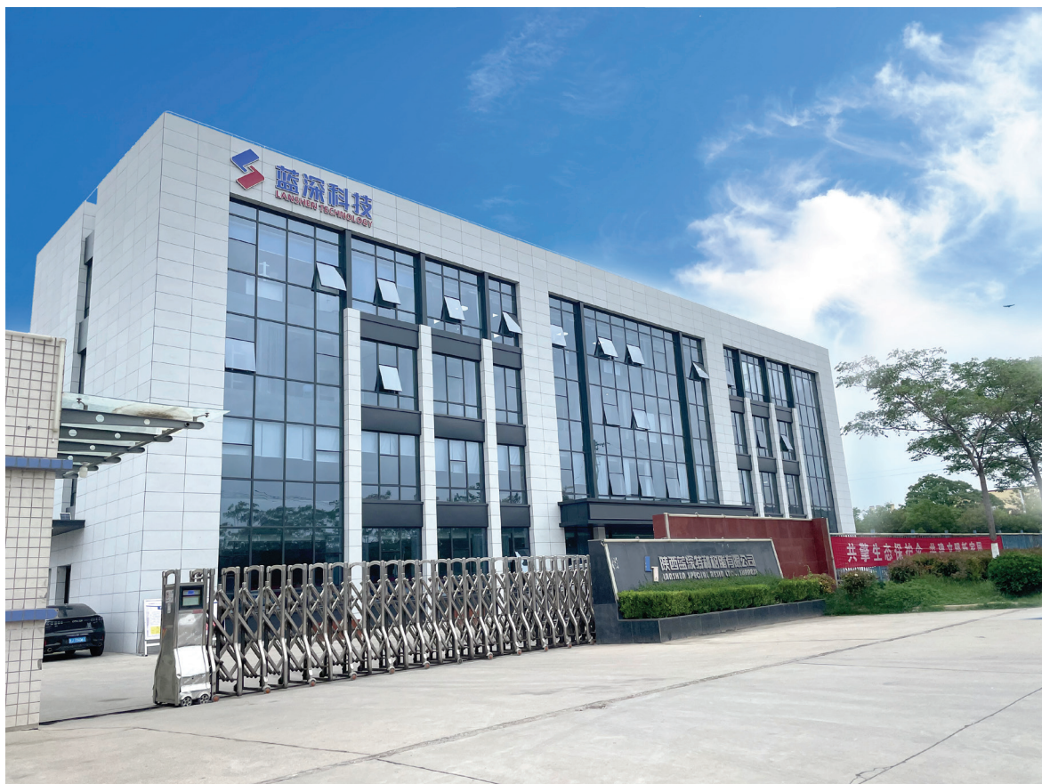
Figure 4: Lanshen Factory, Shaanxi Province, China
