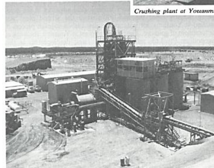
Youanmi Carbon in Leach Gold Plant completed December 1936. (Eastrmet Ltd.)
