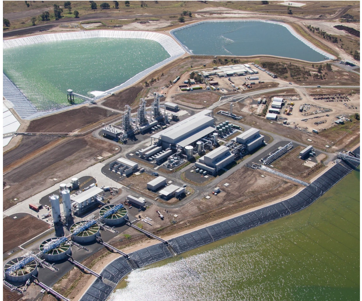
Shell QGC, 100 MLD Northern Water Treatment Plant built by Consortium of GE and Laing O'Rourke. Image courtesy of GE.
