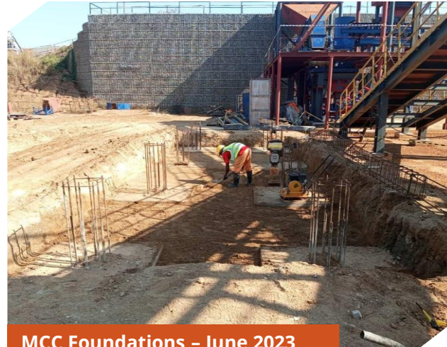
MCC Foundations – June 2023
