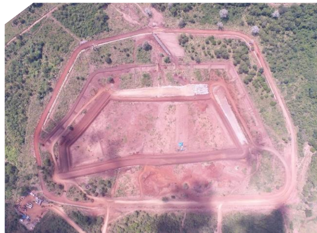
Tailings Storage Facility – May 2023
