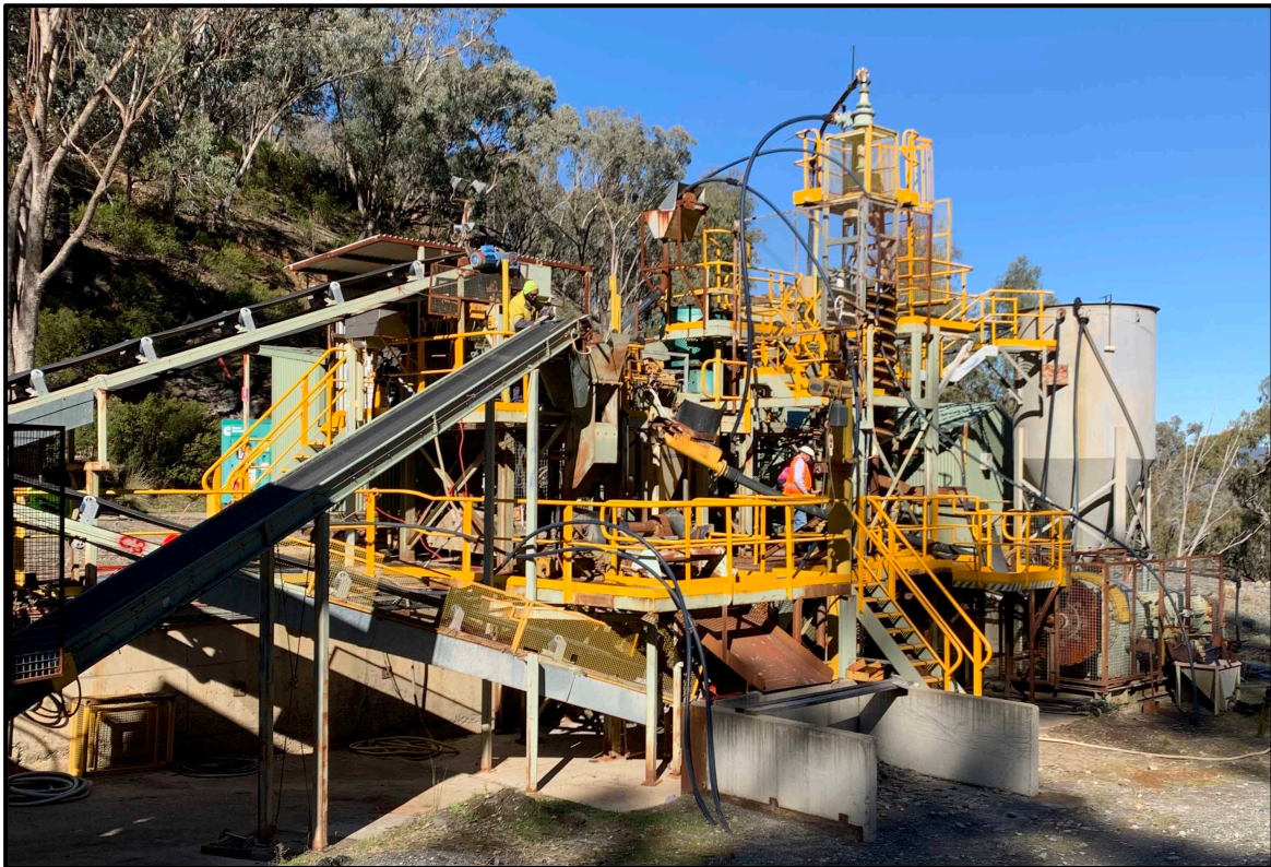
Image 3: Refurbishment work underway at the processing plant
