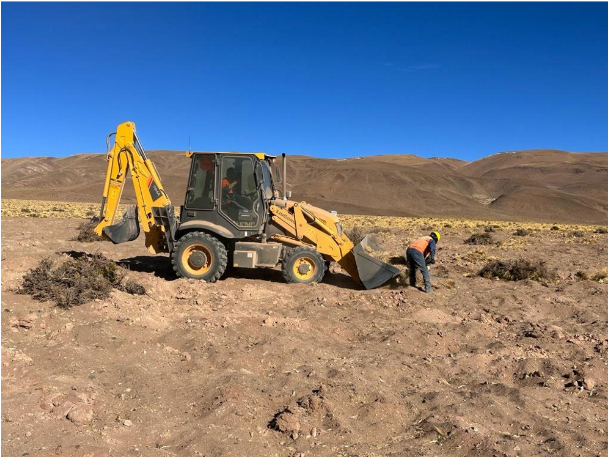
Commencement of top-soil removal at HMW
