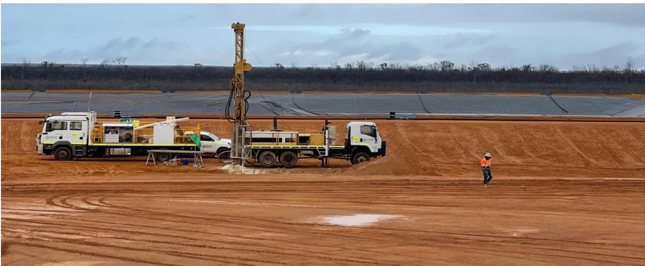
**Figure 2 TSF Piezometer Installation And Drilling**
