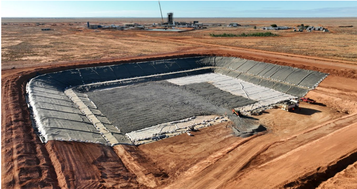
Image 2: 25,000-ton gypsum pond lining being installed
