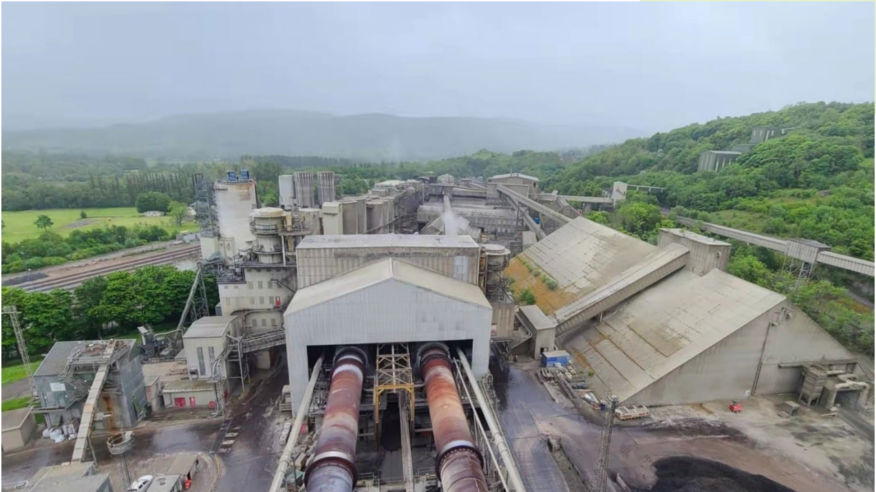
Figure 1 - Breendon Group's Hope Cement Works Facility in Derbyshire, United Kingdom.
