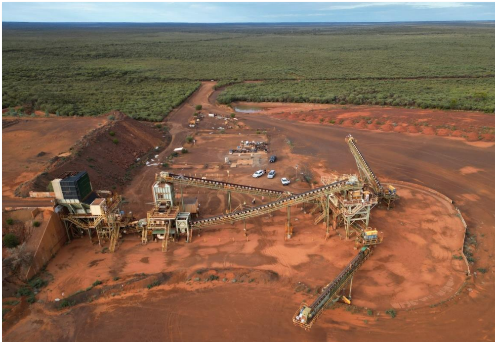
Image 8: Extension Hill crushing and screening plant
