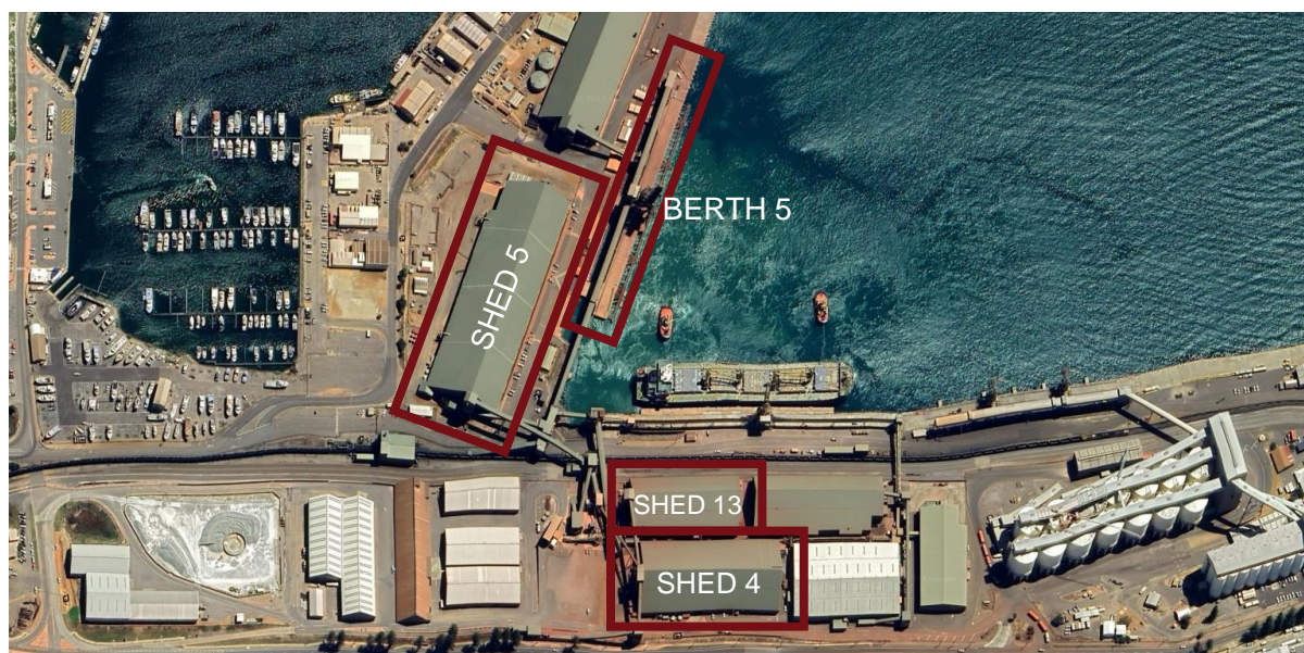
Image 5: Geraldton Port showing Storage Sheds and Road and Rail access
