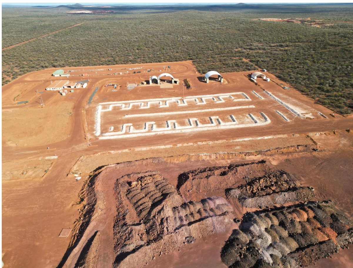
Image 4: Shine Mine Infrastructure, Staging Area, and Ore Stockpiles
