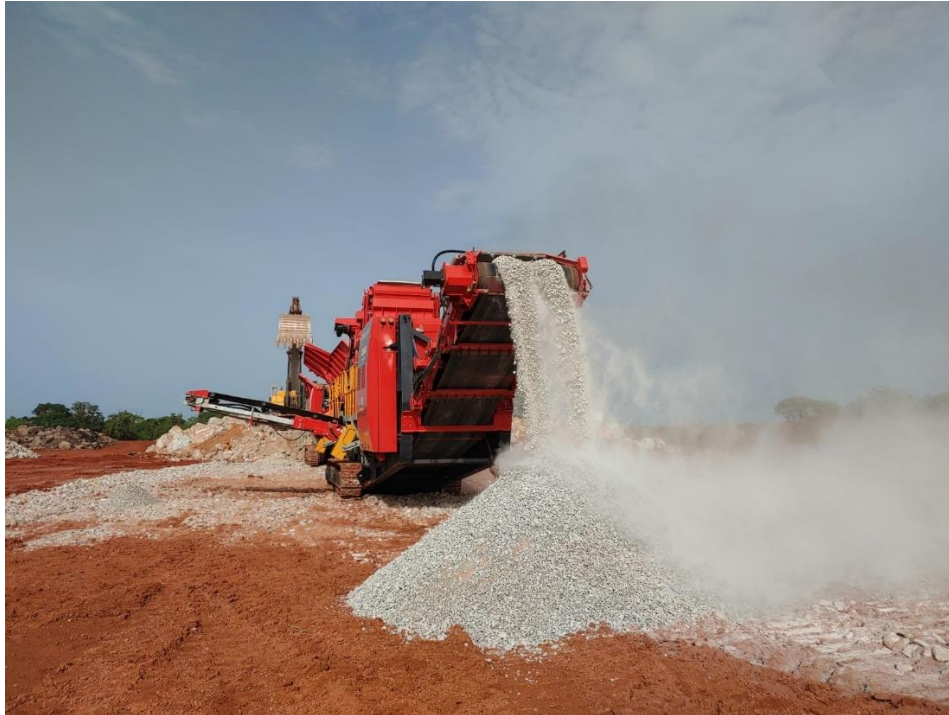
DSO crushing in action at Goulamina.
