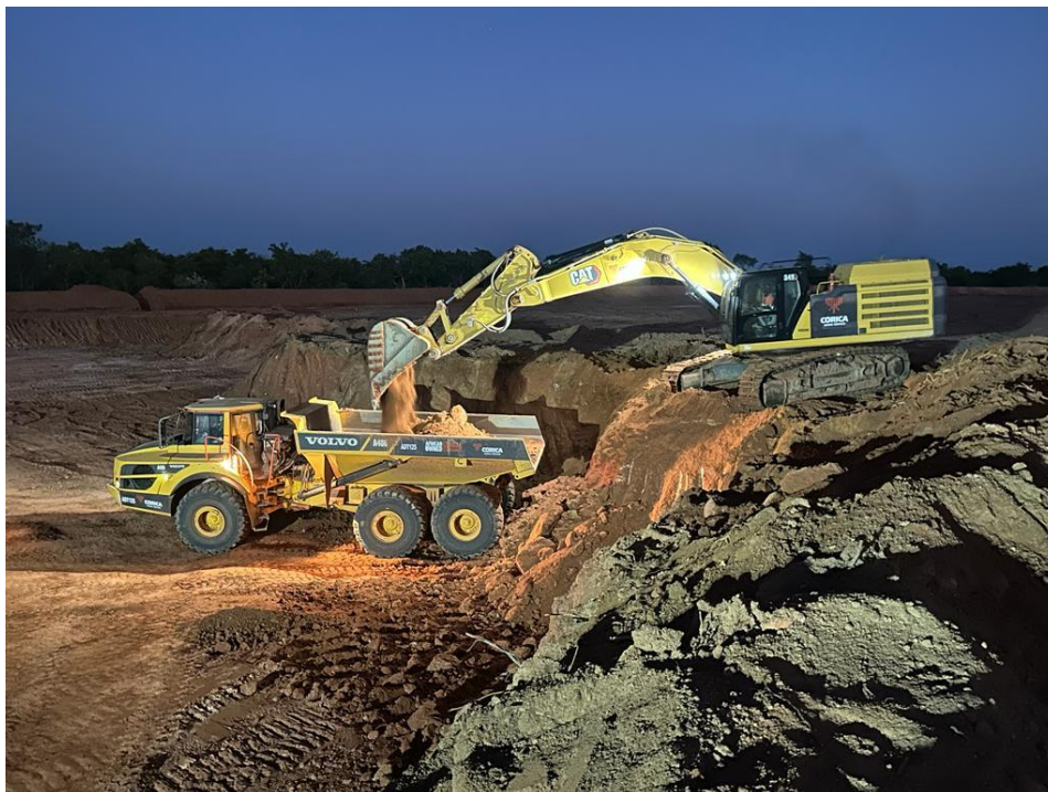
Excavation of the starter pit for DSO at Goulamina.
