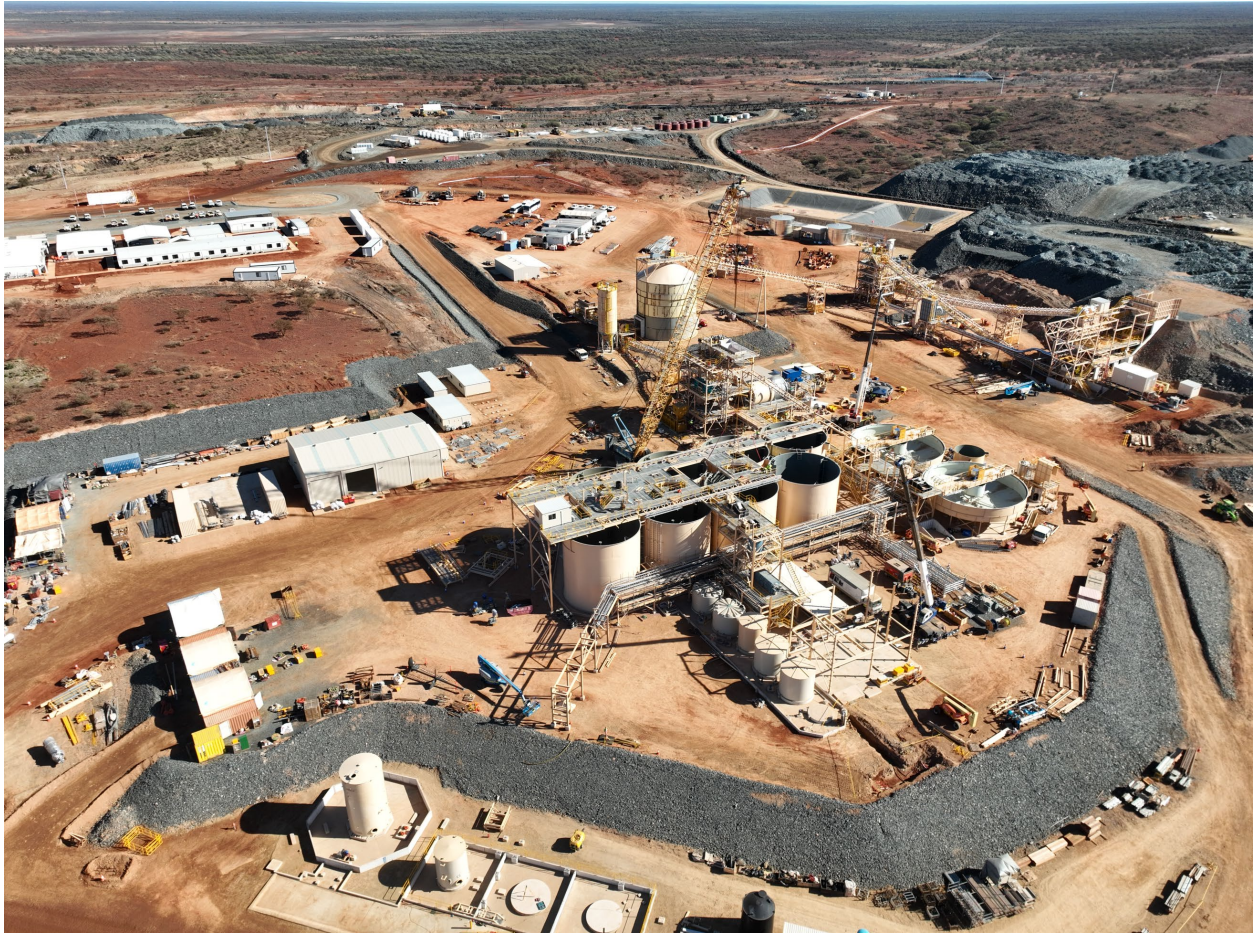
Figure 3: Processing plant construction as at 2 July 2023.
