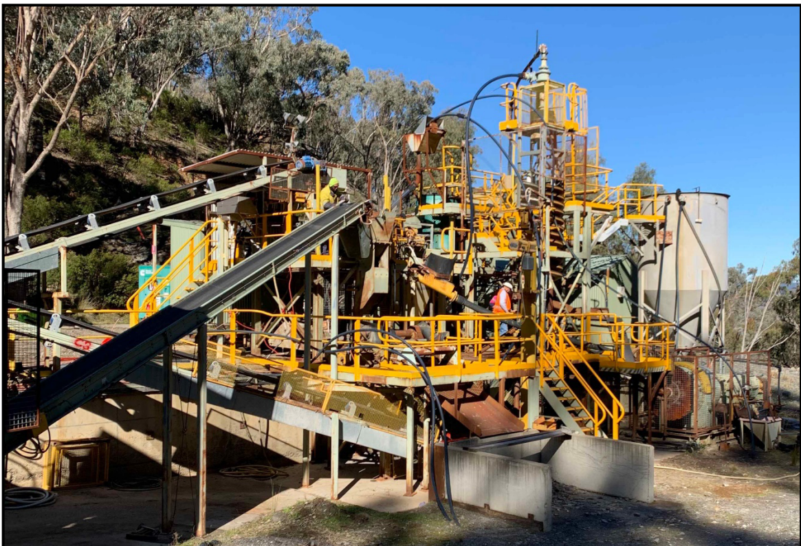
Image 2: Refurbishment work underway at the processing plant
